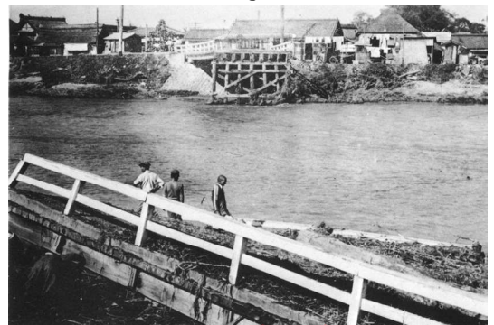
昭和 10 年千秋橋水害 1935 (Showa10) Senshu Bridge flood
